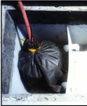
Sump Pump Enclosure & Filter Bag
